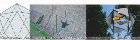
We studied at first different tensecity geometries (cuboctahedron, icosahedron), that focussed our attention, finally choosing the icosahedra, the symmetry of which best fitted with a folding constraint. Then, with bamboos supplied by the Bambouseraie d'Anduze, we have been able to build a tensegrity icosahedron, at the scale of 1/2, with 2,5 to 5 meters long bamboo rods, and we finally achieved a 3D computer drawing of our project
